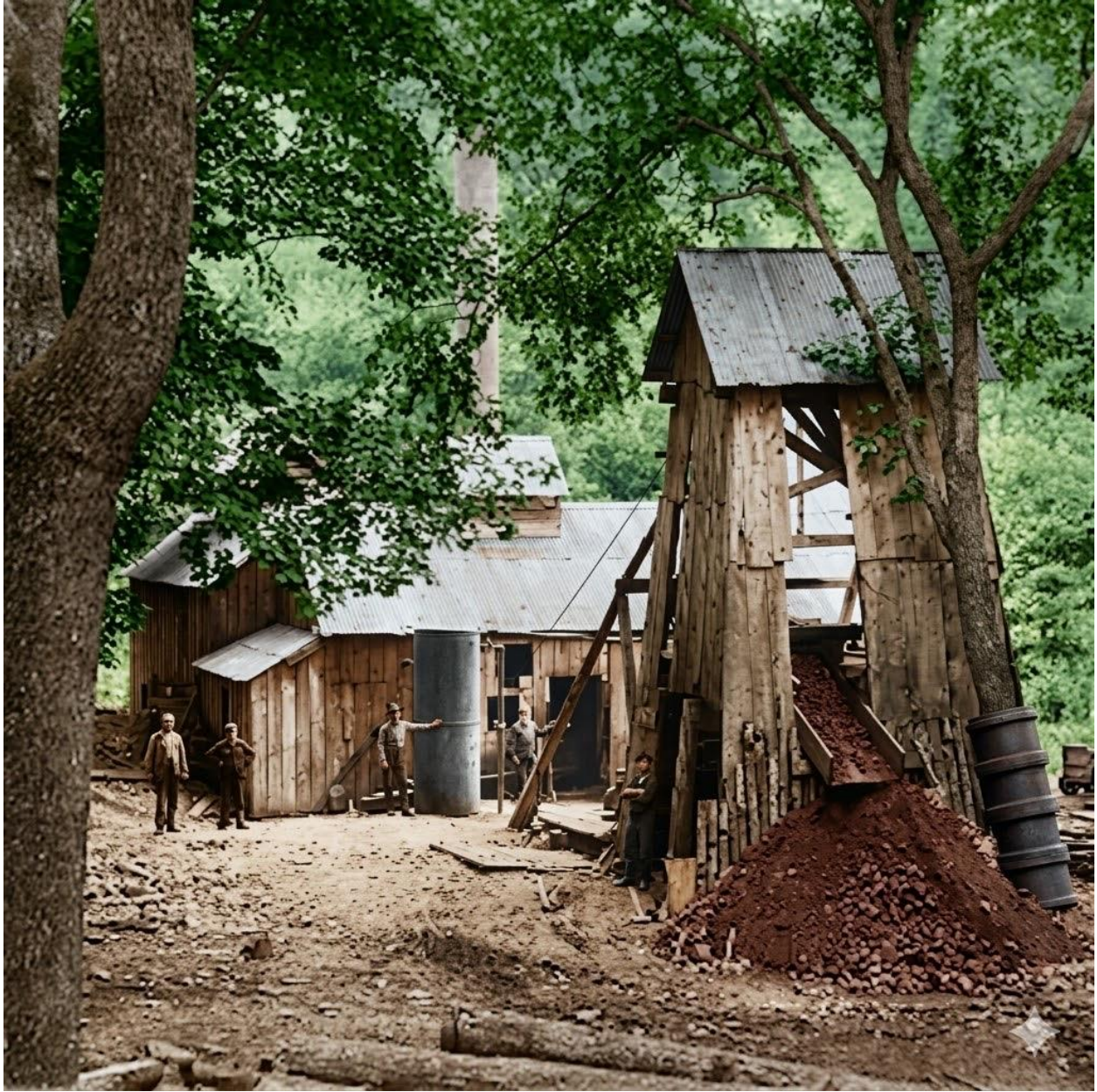
Figure 12. Mine site in Mine Hill Township, Morris County, New Jersey. Courtesy Ferromonte Historical Society. (Ferro monte was Italian for iron mountain). Public domain.
